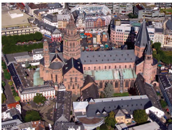
Mainz and its cathedral. Photo: W. Pehlemann 2008
