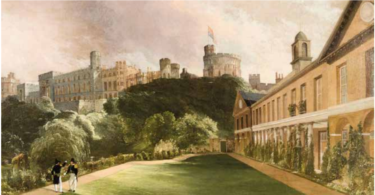
The Naval Knights building at Windsor
