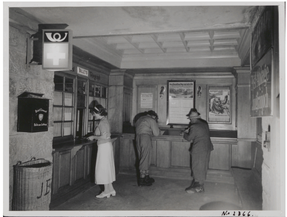
Jungfrauoch post office. The highest post office in Switzerland at 3,460 meters above sea level. It opened on 1 August 1912, together with the railway connection. The historical photo of the counter hall is from the period 1930-1940. Photo: PTT-Archiv
